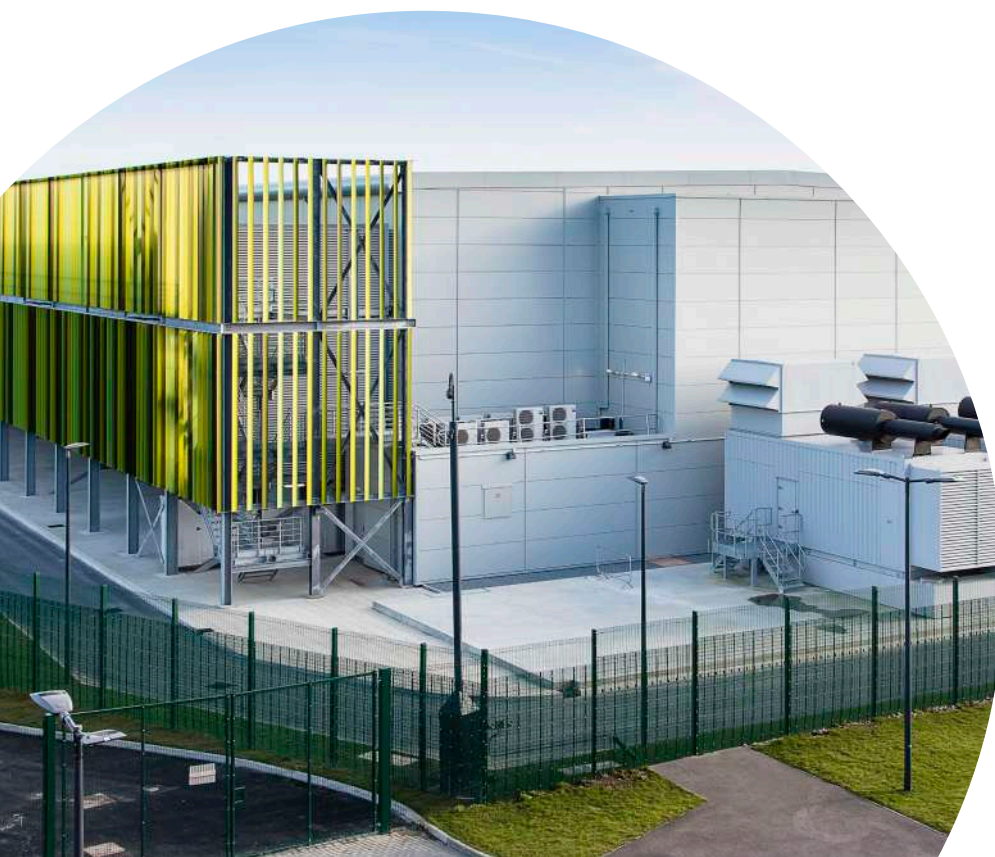
Kao Data's KOLON-01 data center (Harlow) is home to the UK's fastest and most powerful supercomputer, NVIDIA's Cambridge-1. Picture Credit: Kao Data
